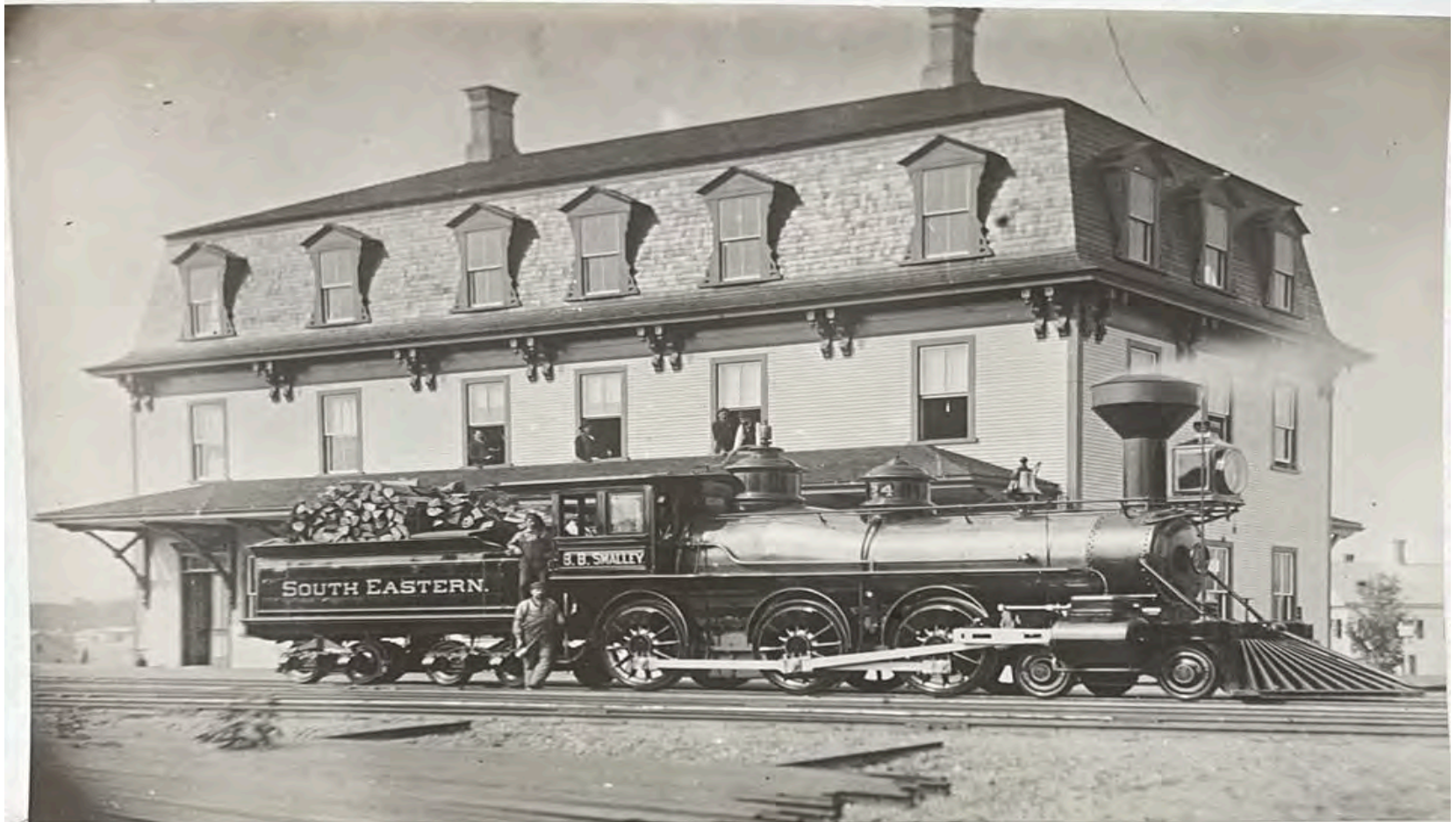
Passenger Station and Superintendent's Office South Eastern R'y, Richford, Vt.
